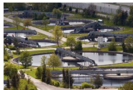
Figure 2 Water treatment plants use chemical treatments, such as adding lime, to precipitate out metal compounds which can then be removed by filtering
