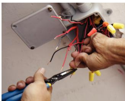
Figure 2 Copper is particularly useful because it is such a good conductor of electricity
