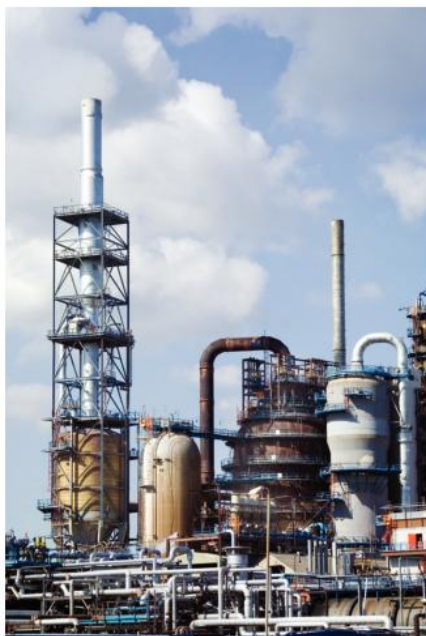
Figure 1 In an oil refinery, huge crackers like this are used to break down large hydrocarbon molecules into smaller ones
