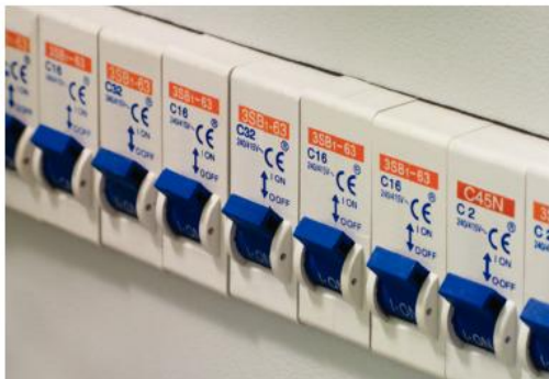
Figure 3 A set of circuit breakers
