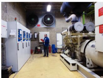
Figure 1 A standby generator
