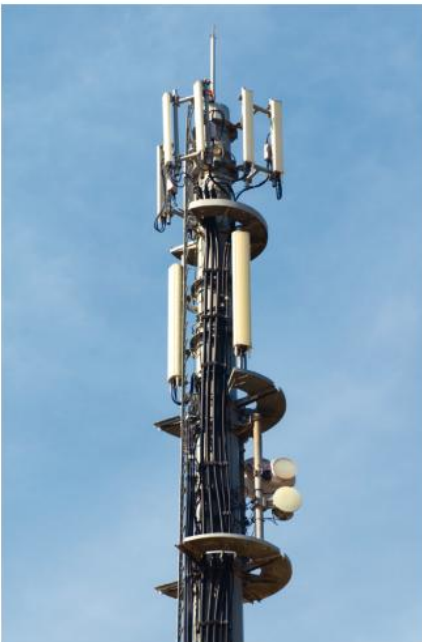
Figure 2 A mobile phone mast
