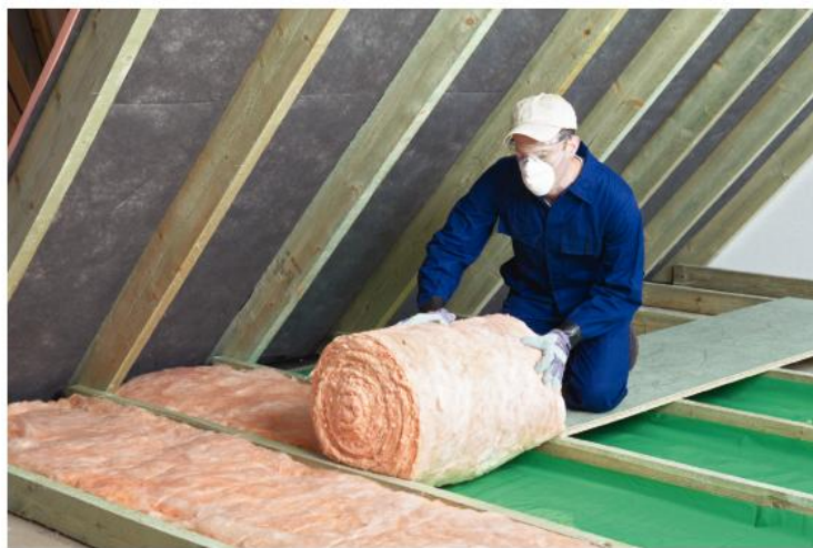
Figure 3 Insulating a loft. The air trapped between fibres make fibreglass a good insulator
