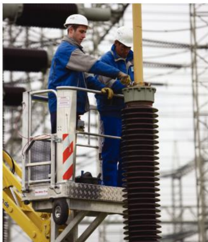
Figure 1 A power transformer under inspection
