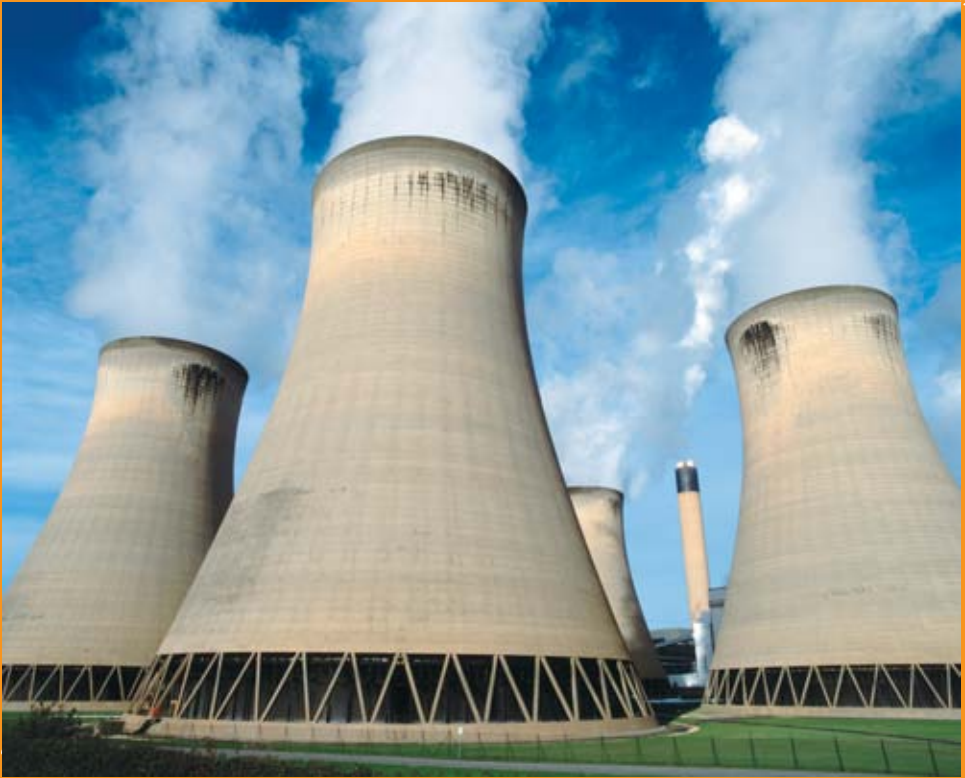
Cooling towers at a power plant.
