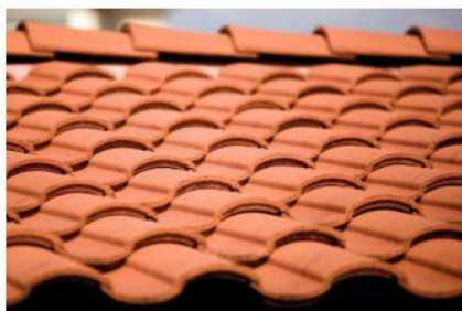
This roof is covered in terracotta tiles
