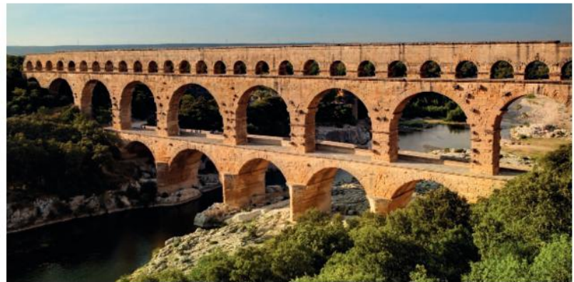
This Roman viaduct in Pont du Gard, France, has stood for 2000 years
