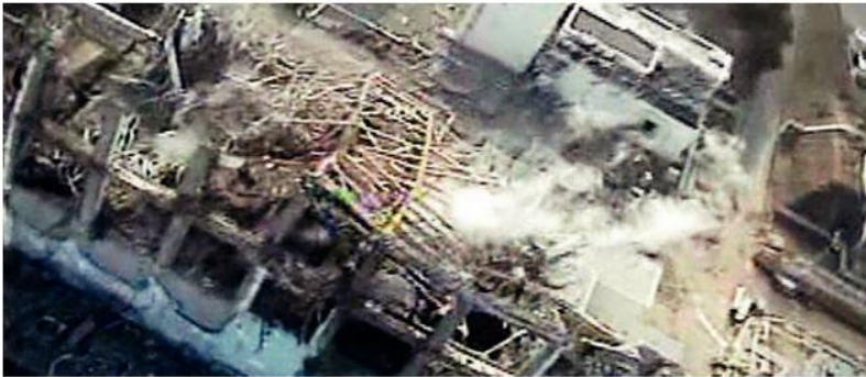
A tsunami in Japan in 2010 damaged the Fukushima nuclear reactors. Hundreds of square kilometres of land had to be evacuated for health and safety reasons
