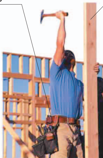
el albañil construction worker
